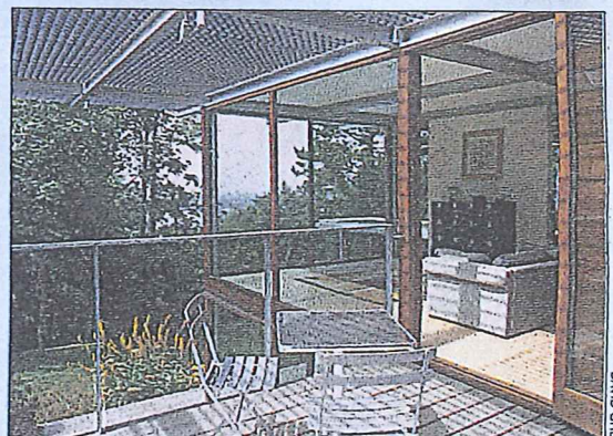
Economy: building costs were kept low by cladding a simple steel frame with timber
